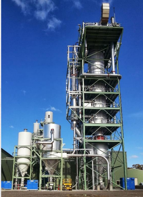
Lixhe, Belgium. LEILAC-project. Funded through H2020 Building pilot for Phase 2 test. Capture 100 000 ton CO 2 / year
