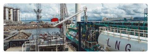
At Øygarden,  ${\rm CO_2}$  is offloaded and stored temporarily in onshore tanks before injection.
